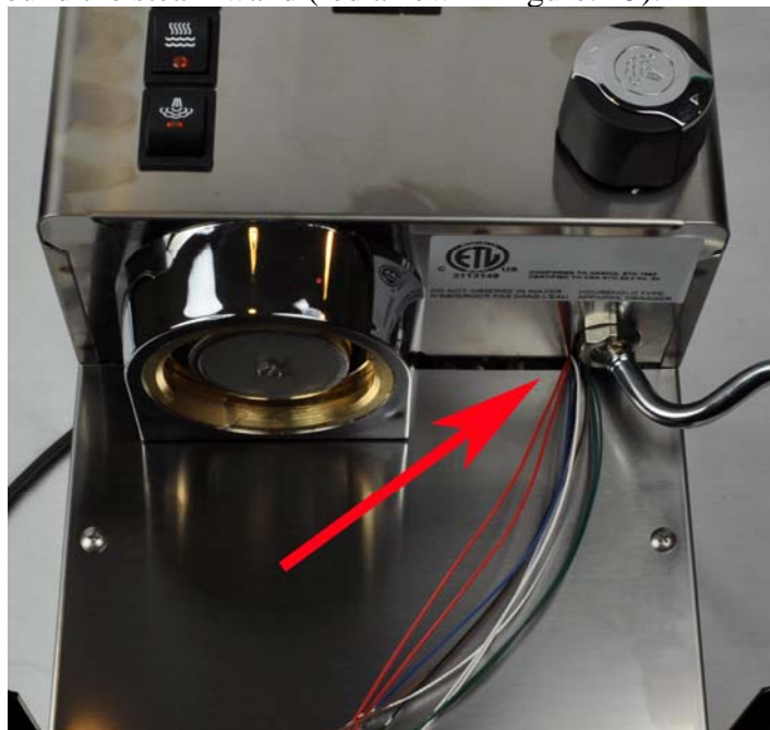
Figure 25. Cables going through the back panel of the controller box.
