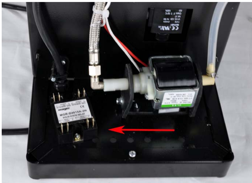
Figure 16a. SSR mounted on the base.
